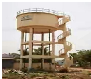
Fig.2 Elevated water tank
