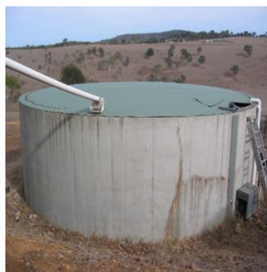
Fig.1 Tanks resting on ground
