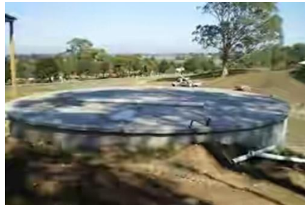
Fig.3 Under ground water tank
